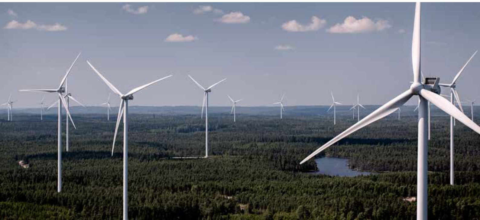
The Lemnhult wind power plant consists of 32 V112-3.0 MW turbines, producing enough electricity to support the residential consumption of 70,000 households in Sweden.
