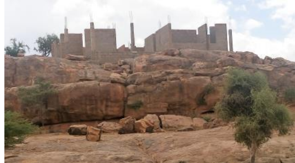
2) Permanent house under construction in Namerei
